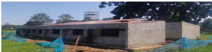
vi) Dispensary roofed to near completion with splash apron construction ongoing
