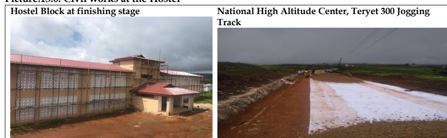
Picture.13.0: Civil works at the Hostel
