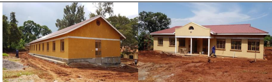
Dormitory block Jinja PTC June 2019
