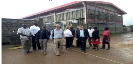
The soon to be commissioned multipurpose workshop at Nakapiripirit Technical Institute
