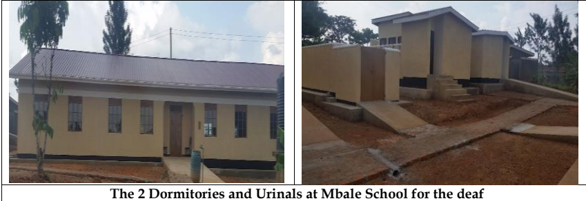
Picture.15.0: Facilities constructed at Mbale School for the deaf
